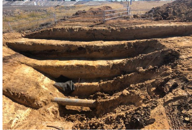
A pipeline dig-up which is required when an in-line inspection identifies some potential coating or corrosion issues
